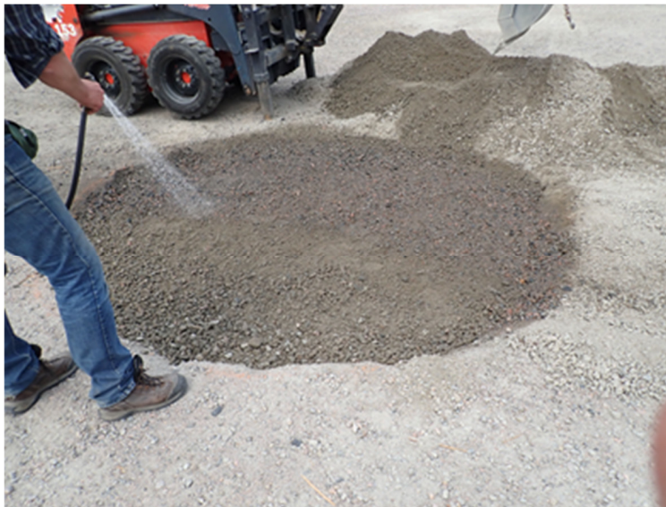
Figure 1: Adding water to the soil during a test site preparation.
