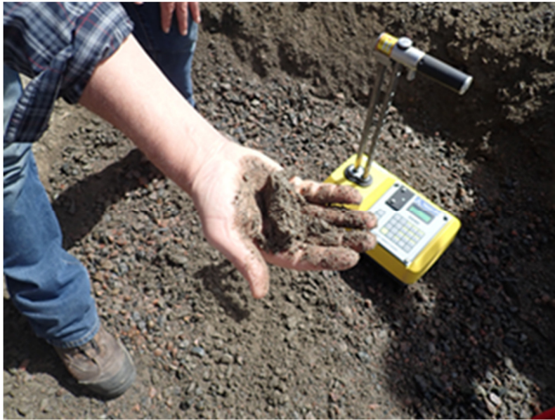
Figure 16: Assessment of the moisture content using the touch and feel method.
