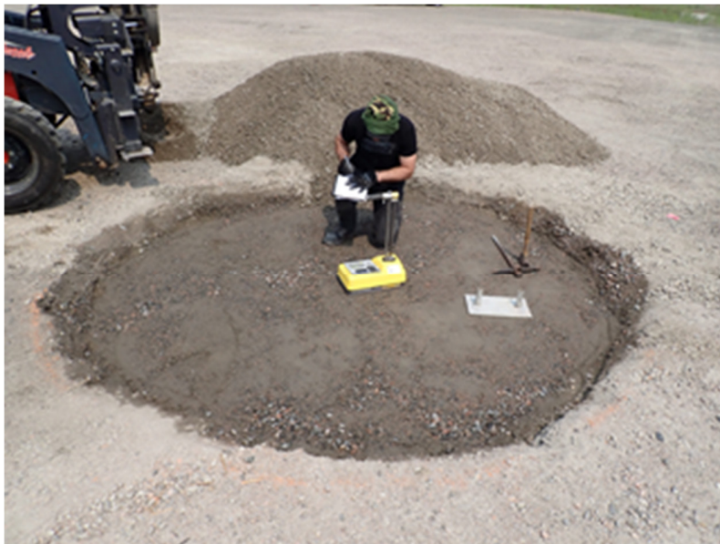
Figure 17: Measurement of the soil conditions using the nuclear method [5].
