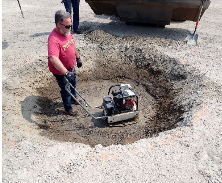
Figure 18: Compaction of the soil using as small vibrating plate compactor.
