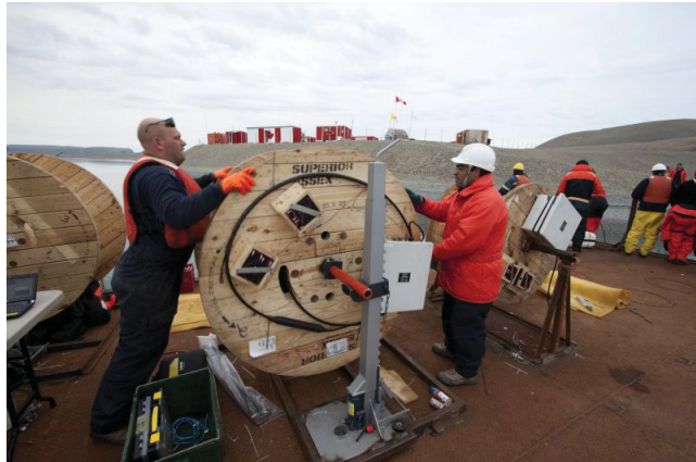
Figure 7. Telemetry cable deployment.
