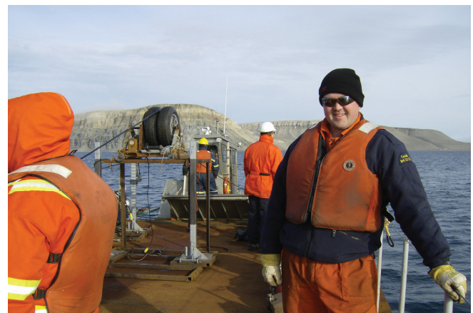
Figure 9. Using the mule to under-run an array cable.
