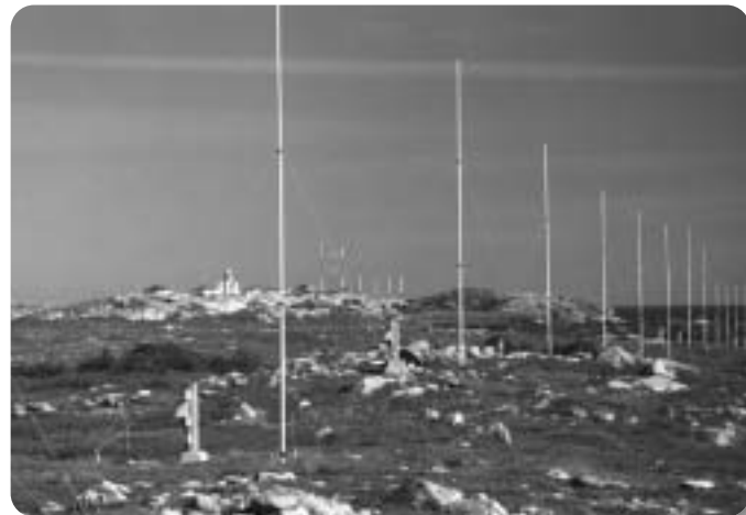
High Frequency Surface Wave Radar Installation in Newfoundland
