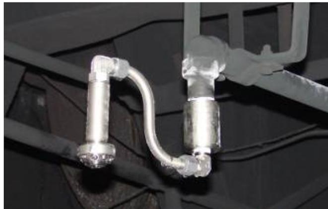
*Figure A-8. Securiplex Water Mist Nozzle in Machinery Space*
