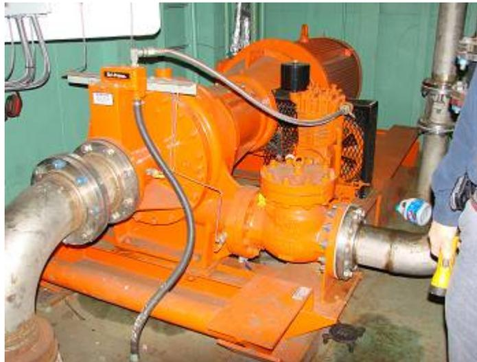
**Figure A-14. LPD-17 Firemain/Water Mist Pump (ex-USS Shadwell)**
