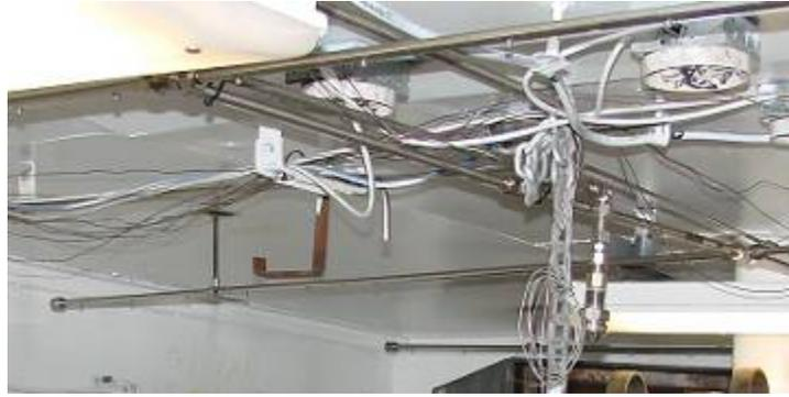
**Figure A-9. Water Mist Nozzles - Electronic Space**
