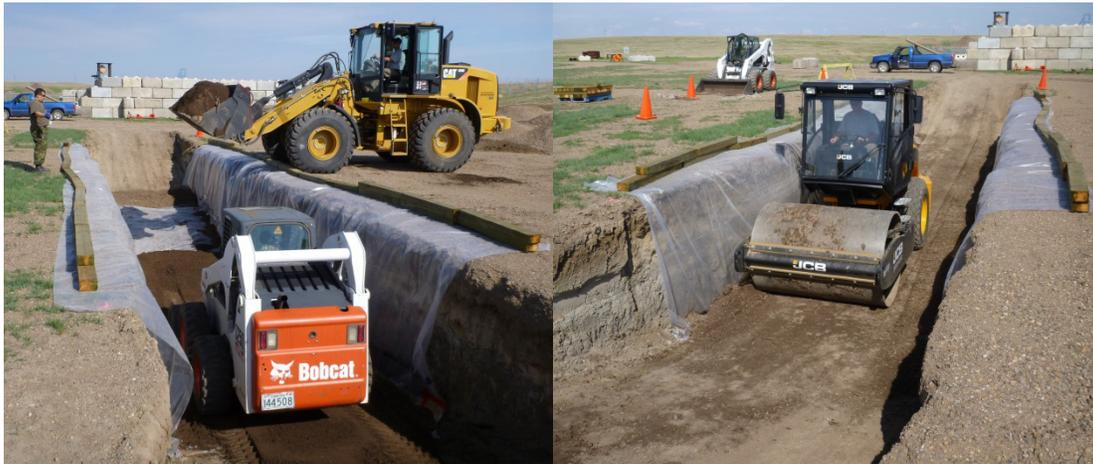
Figure 2: Test pit construction
