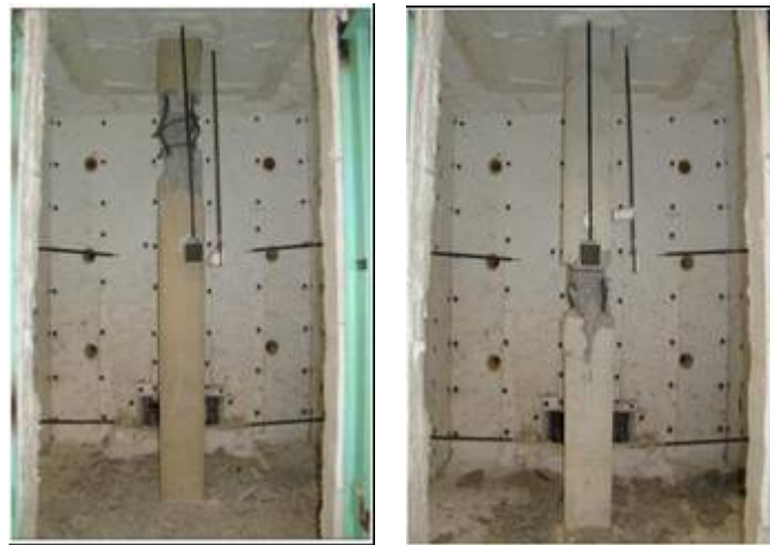
Figure 11. The two column specimens after testing for failure loads; column tested for E1529 on the left and column tested for E119 on the right.
